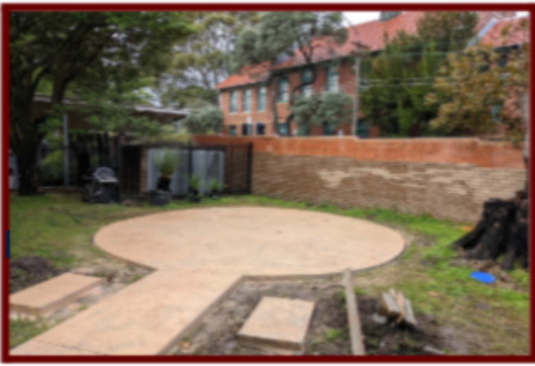
Concrete has been poured in Koori Garden ready for sandstone seating
